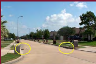
Storm sewers in Spencer Landing
