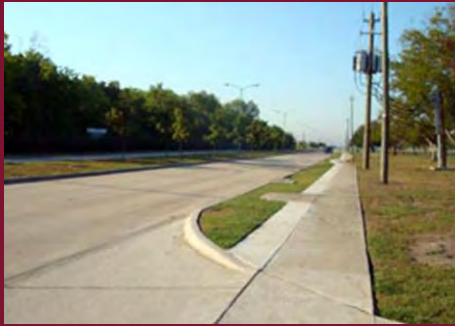
Sidewalk Expansion Retrofit
