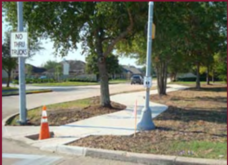
New Sidewalk Construction
