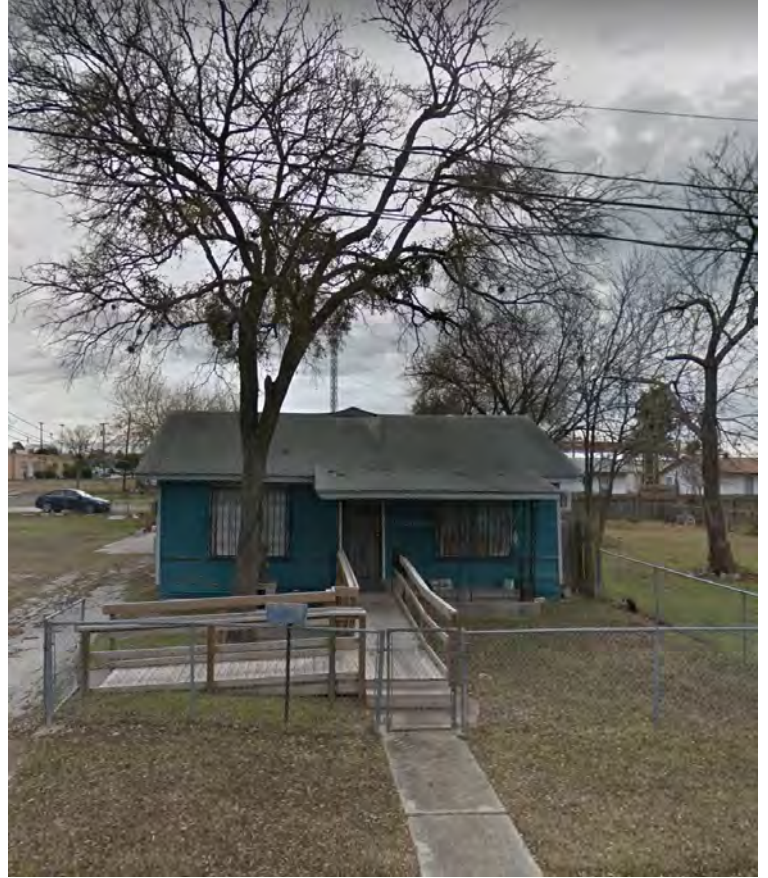
Potential Blight #6: Home in need of maintenance on Milliard St.
