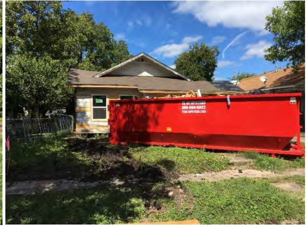
B. 215 W. High Ave. (remodel in progress)
