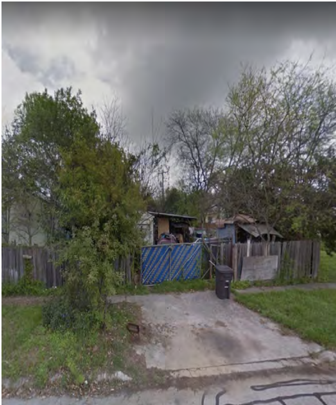
Potential Blight #1: Home in need of maintenance on Breeden St.
