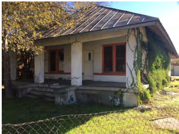
B. 1442 Division Ave. Vacant house next to Pan American Restaurant
