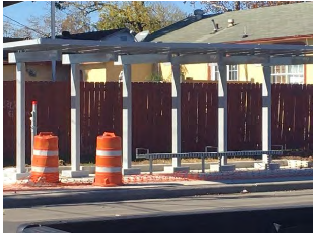
I. New bus stop with covered seating
