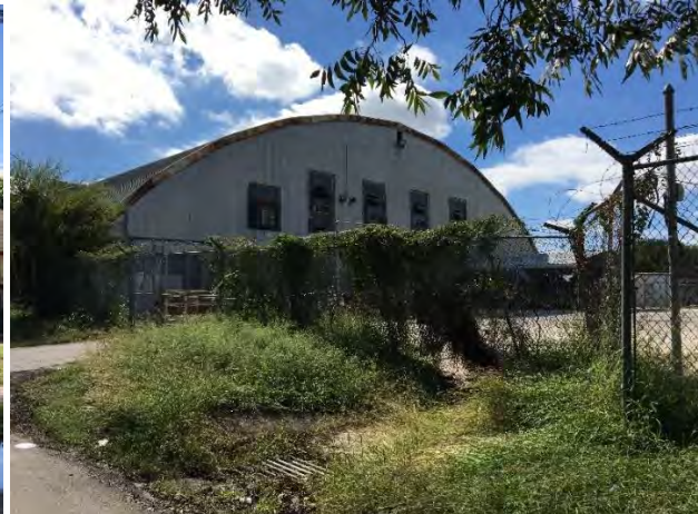
D. 211 W. Drexel Ave. (SAISD storage building)
