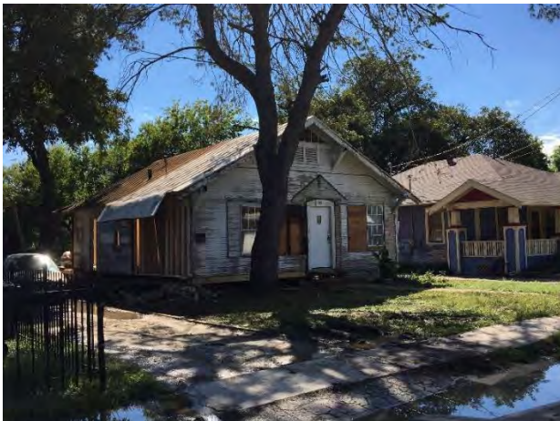
C. 510 W. Drexel Ave. (remodel in progress)
