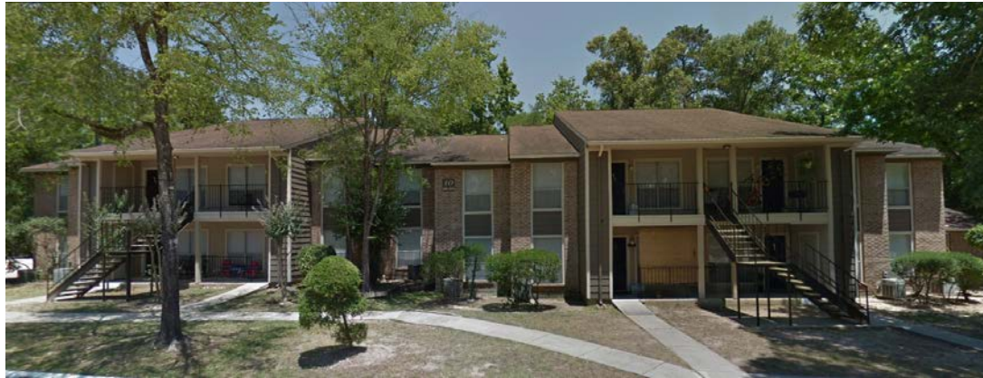
TYPICAL BUILDING ELEVATION/PHOTO
