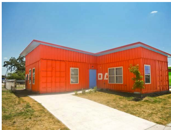
A house built using three 45-foot shipping containers is part of a comparable study on energy efficiency funded by the Neighborhood Stabilization Program (Photo: SAAHC)
