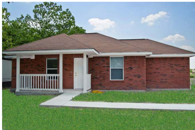
HOME's Homeowner Rehabilitation Assistance Program helps replace homes that have become uninhabitable.
