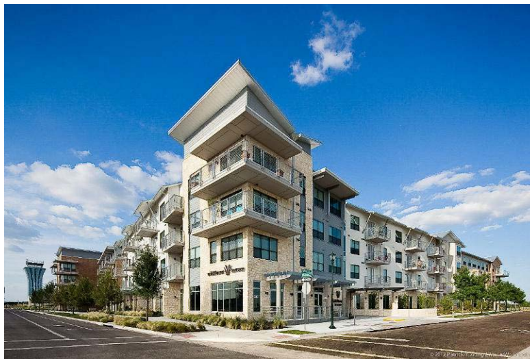
The Multifamily Finance Production's Housing Tax Credit Program provided funding for the development of Wildflower Terrace (Photo: Patrick Y. Wong)
