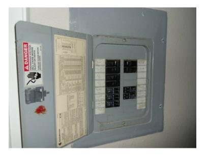
30. Electrical branch wiring in the buildings is copper, and the circuit breakers in the electrical subpanels are properly labeled.
