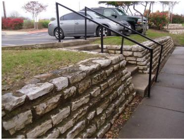
38. Mortared stone retaining walls on the site are in average to good condition.
