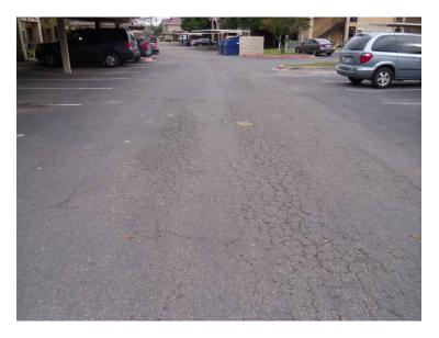
43. Some of the asphalt pavement is showing evidence of stress and deterioration. Note the crack blocking asphalt pavement in this photo.
