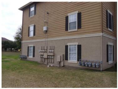
41. The view of the end elevation of a building shows electrical and natural gas connections, and electric disconnects and meters.
