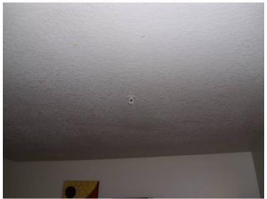
29. Buildings 2, 3, 5, 11, and 13 are three-story buildings that contain fire suppression systems. Shown is a typical pendant type sprinkler head on the ceiling of the bedroom in this apartment.
