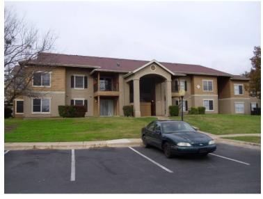
8. The apartment buildings on the site are two and three-stories in height. The buildings have pitched roofs and slab on grade foundations.
