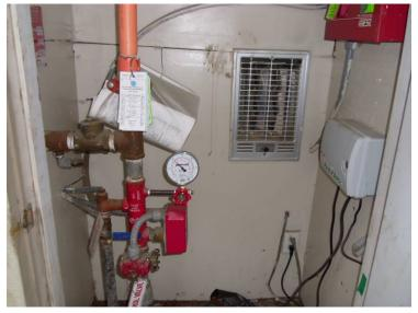
35. This is a view of a typical fire riser closet in buildings 2, 3, 5, 11, and 13. All code required components are present.
