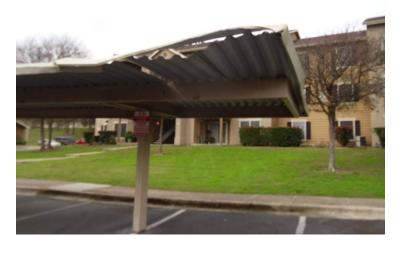
45. Vehicular damage was observed on at least six carports that need immediate repair.
