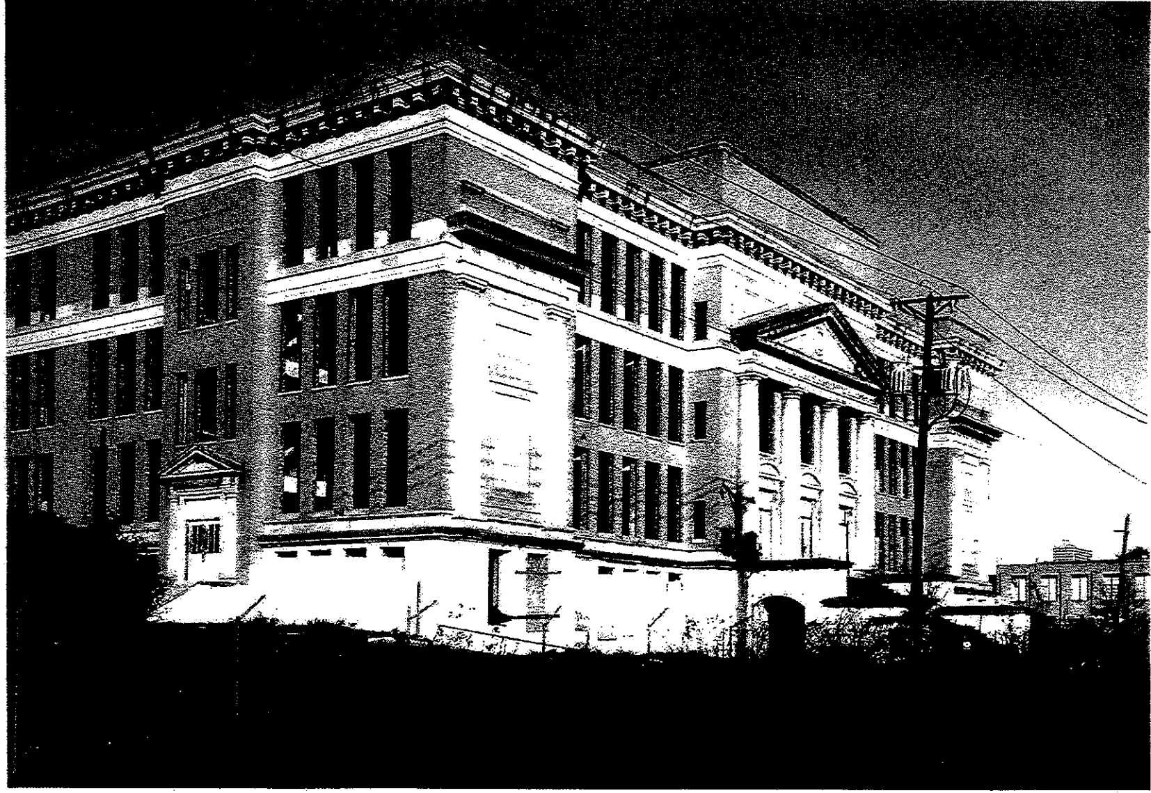
NPS-4005 Fort Worth High School 1015 South Jennings Avenue Fort Worth, Texas 76104 Part 2&3, photographs, 1/1/5/01
