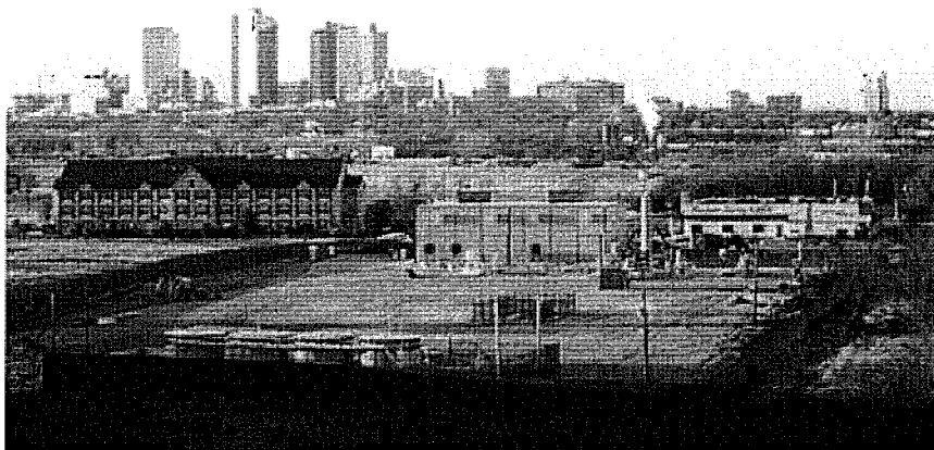
The Mercado Compressor Station does not disturb a hotel in Fort Worth.
