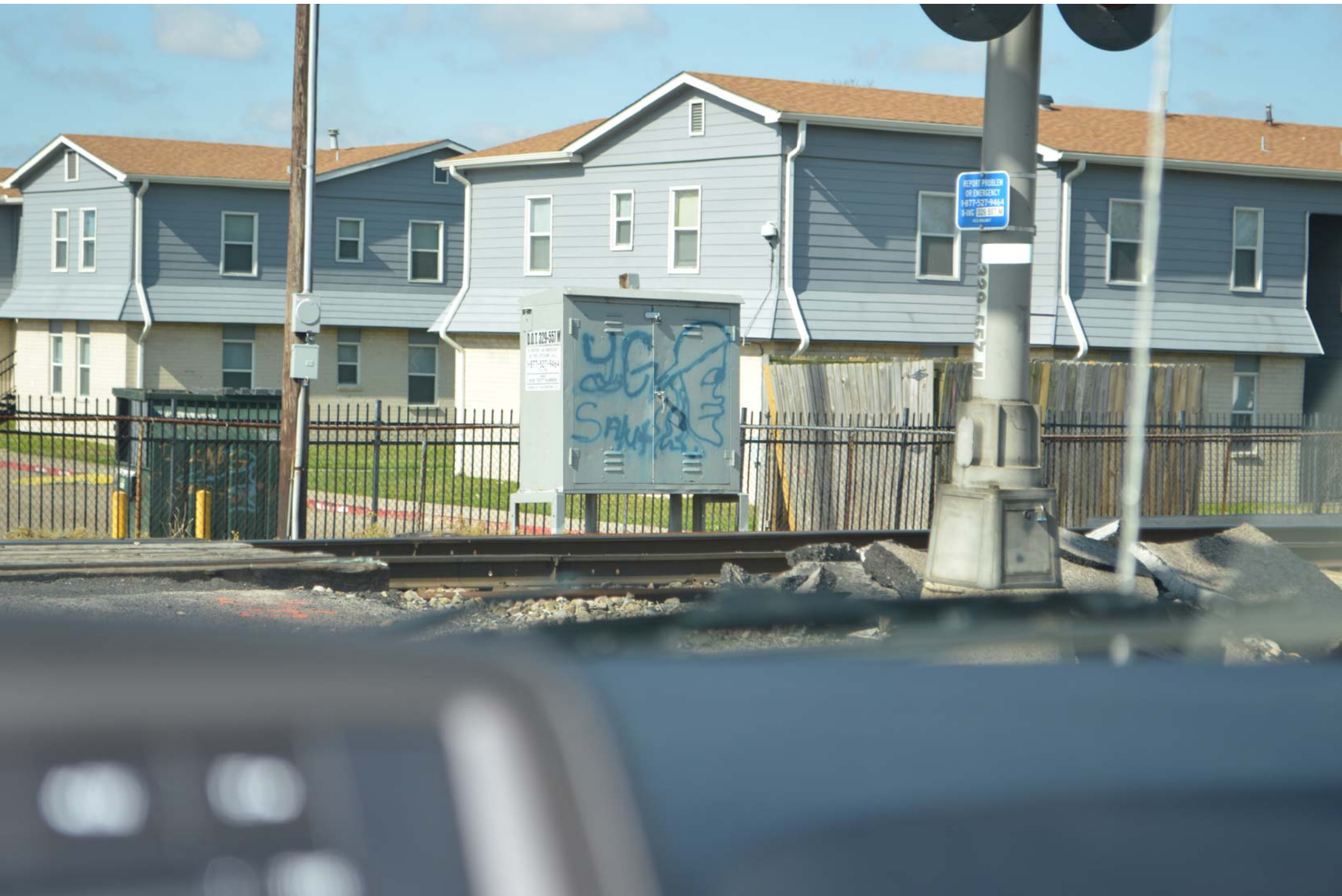
taken from southern corner of site
