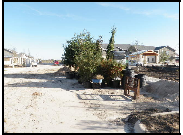
6. Landscaping materials were stored adjacent central park.
