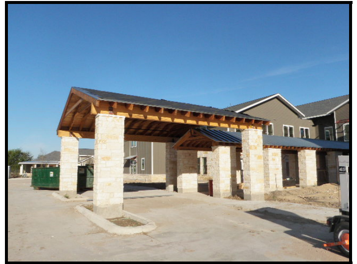
14. Exterior finishes/roofing was complete at Building 1A/B.
