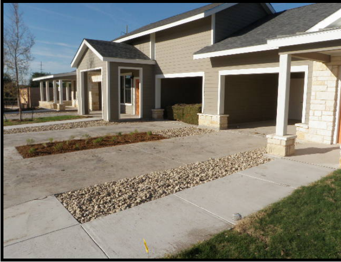
5. Exterior finishes were substantially complete at Building 3.
