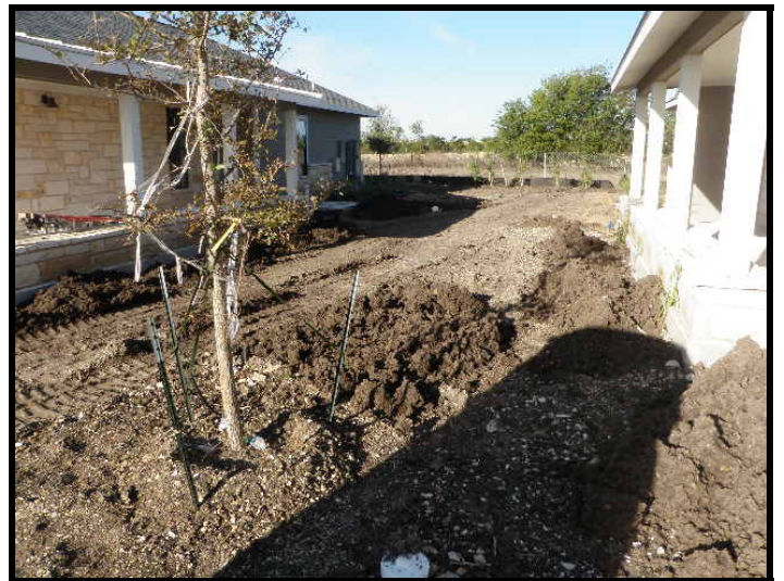
4. Landscaping was in progress adjacent Building 2.
