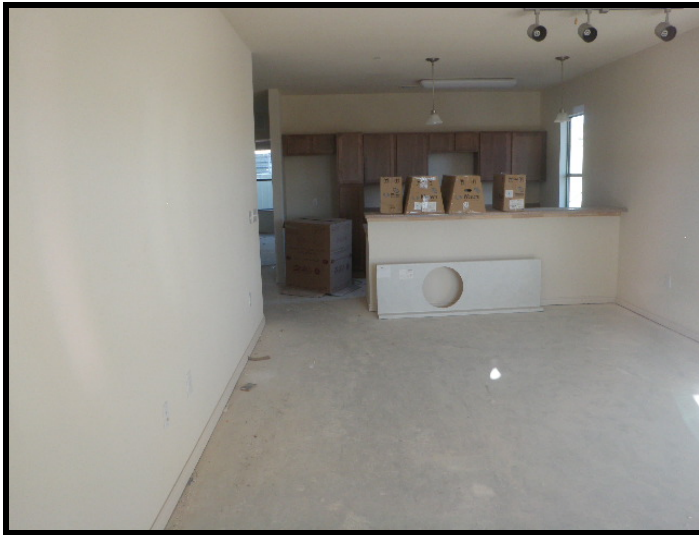
1. Flooring remains to be accomplished at Building 2.
