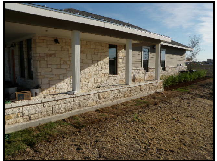
12. Exterior finishes were substantially complete at Building 6.
