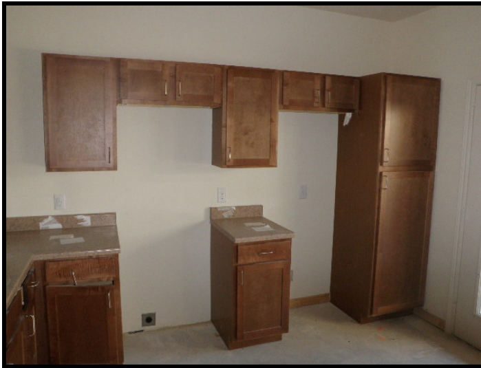
9. Cabinets and countertops have been installed at Building 5.
