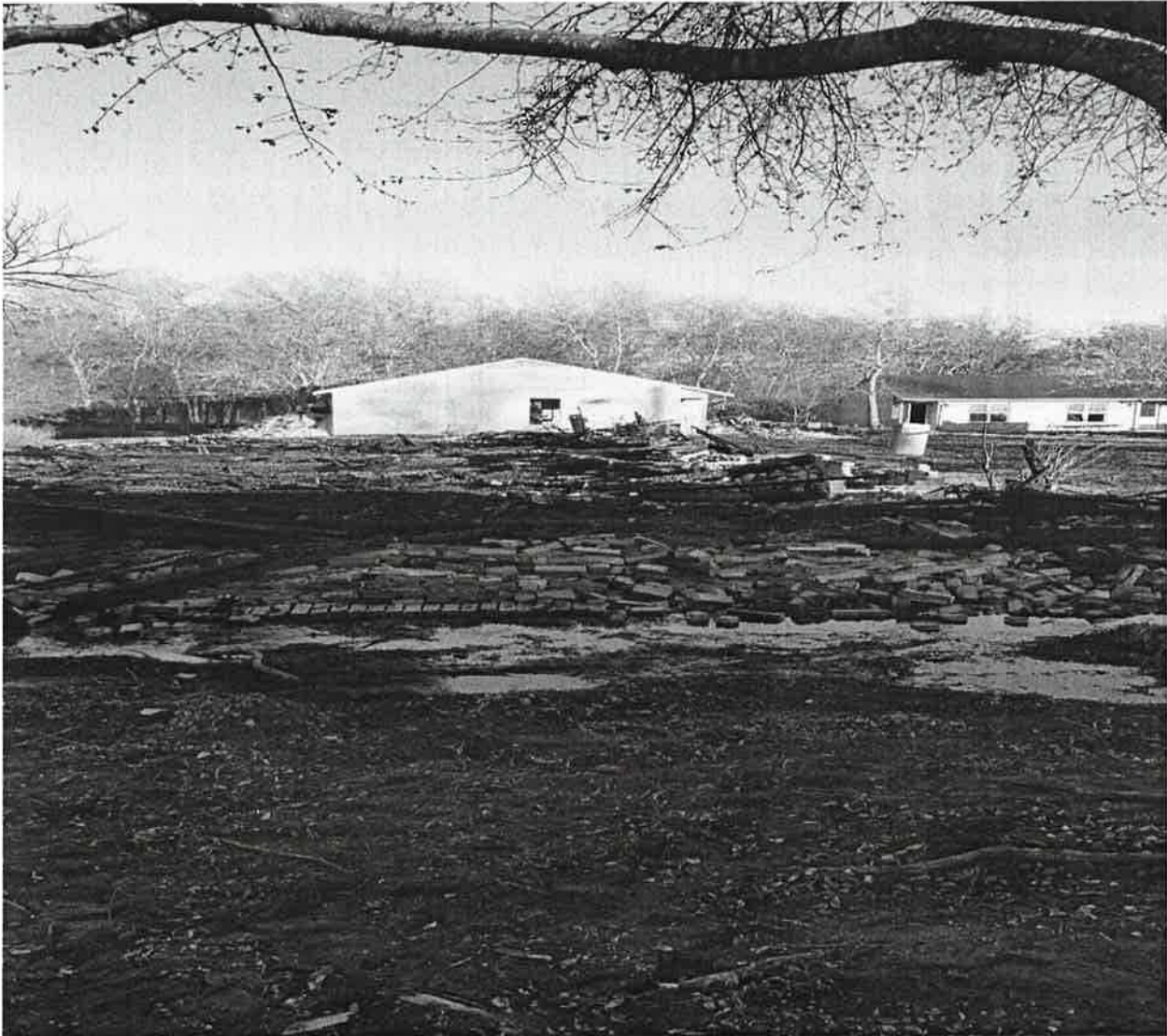
Building Four (4) Fire debris.
