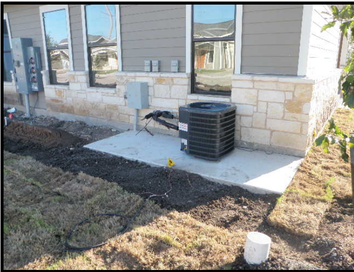
7. Grade mounted condensing unit installation was in progress at Building 4.
