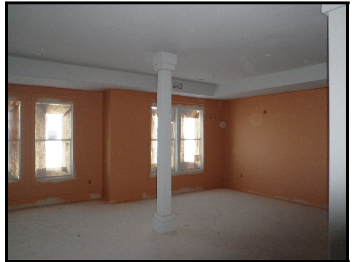
16. Interior paint was nearing completion at east portion of Building 1A/B.
