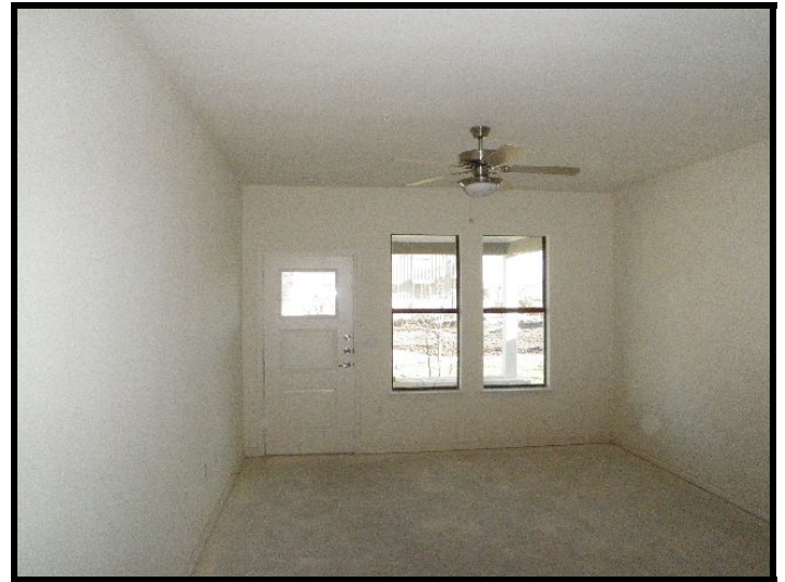
10. Interior fixtures and finishes were complete at Building 5.
