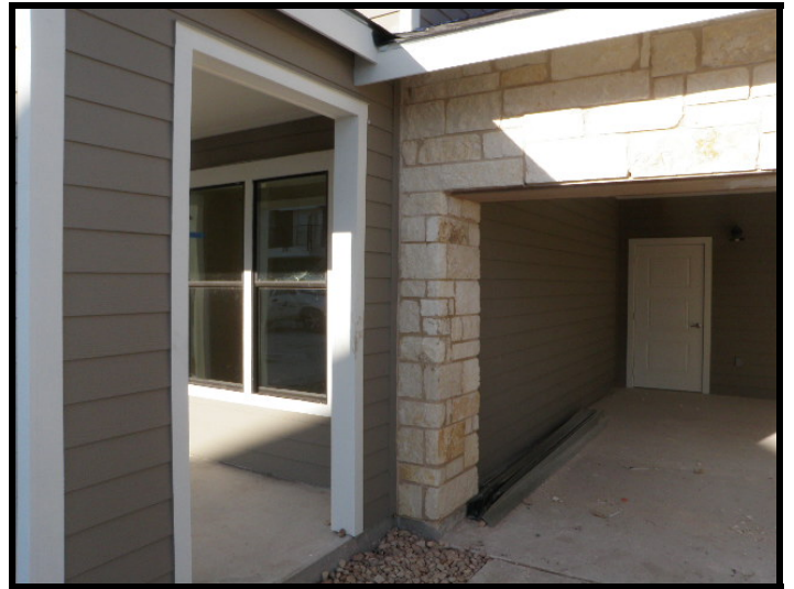
2. Exterior finishes including stone and siding have been completed at Building 2.
