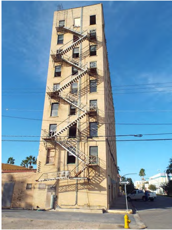
Building façade w/ exterior fire escape – south elevation.
