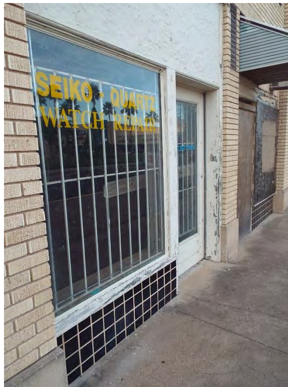
Existing storefront between pilaster 2 and 3 of east façade.
