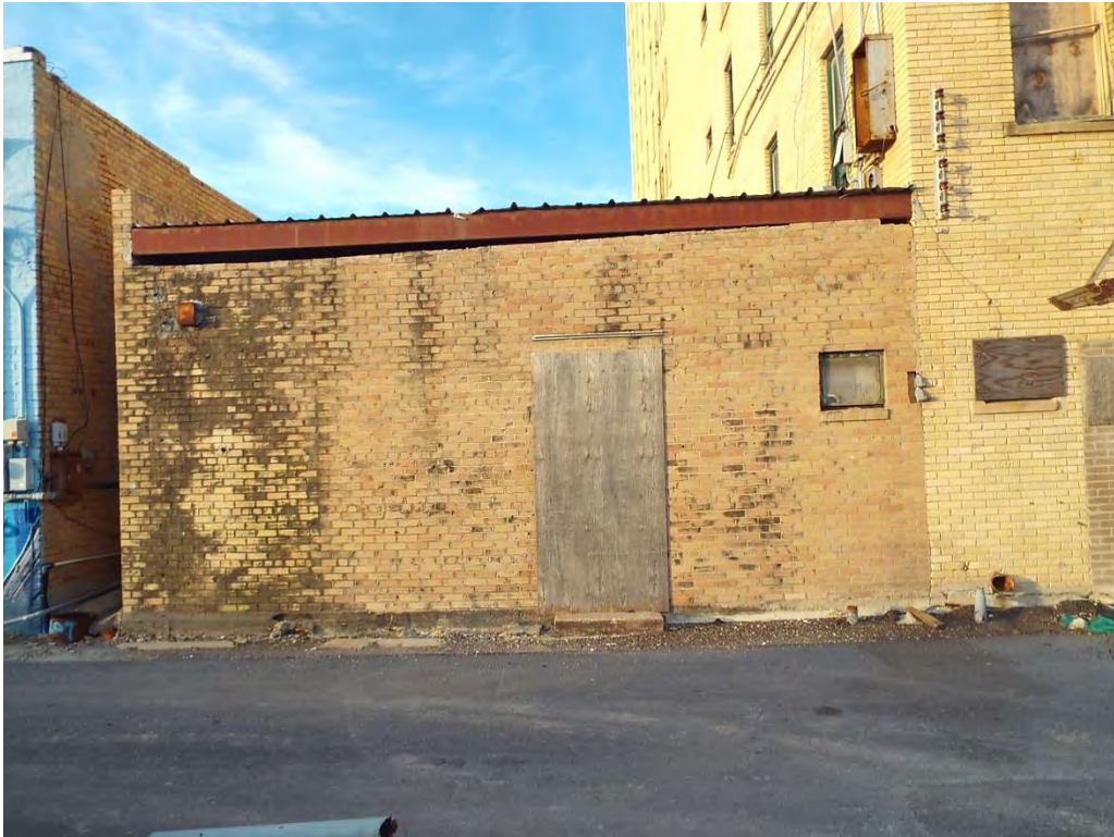
Single storey building to west of main building – south elevation.
