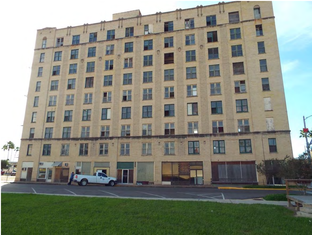
Building façade – looking west across S. A St.
