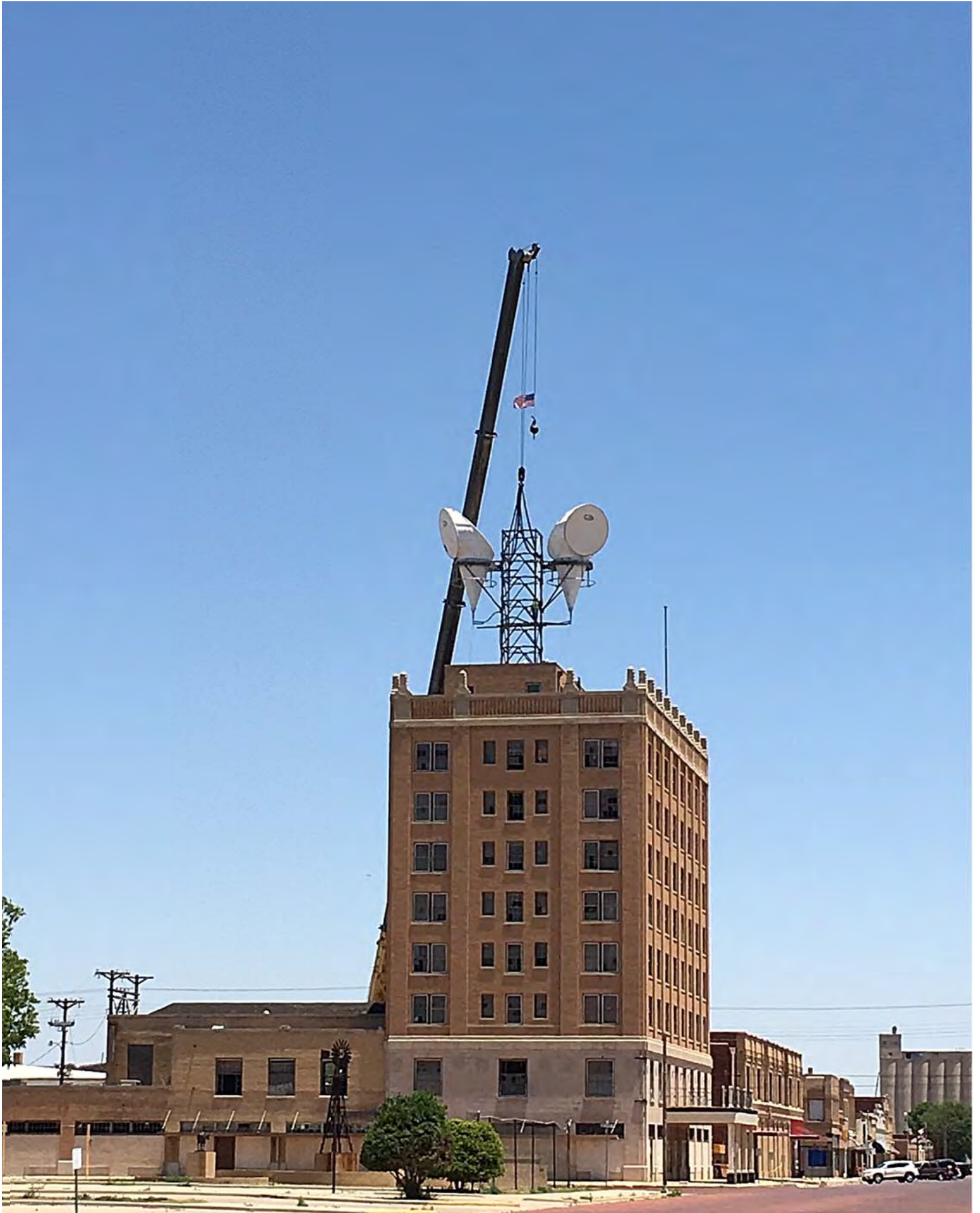
16034 Conrad Lofts, Plainview, Texas Under Construction (2016 HTC Award, MRE Capital)
