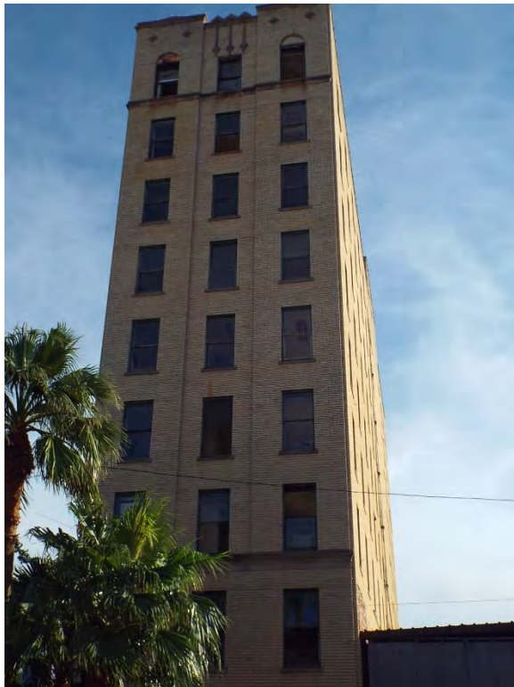
Building façade – 2 nd – 9 th floors – west elevation.
