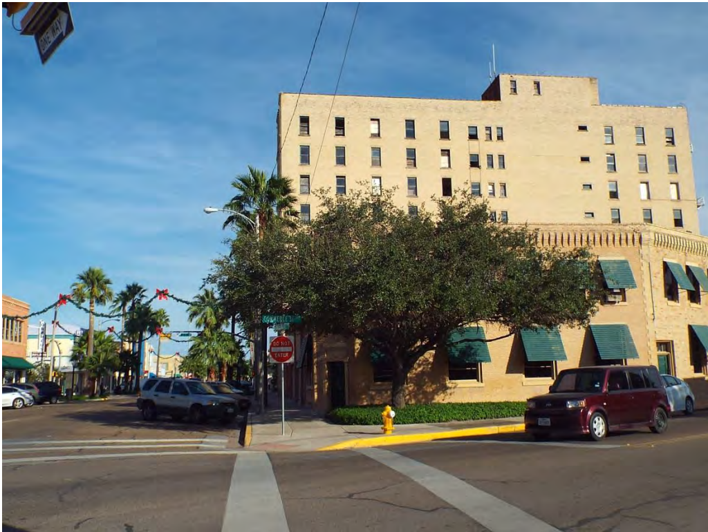
Building façade from South Commerce St. – west elevation.
