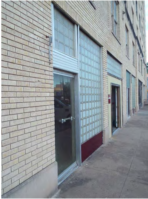
Existing storefront between pilaster 3 and 4 of east façade.
