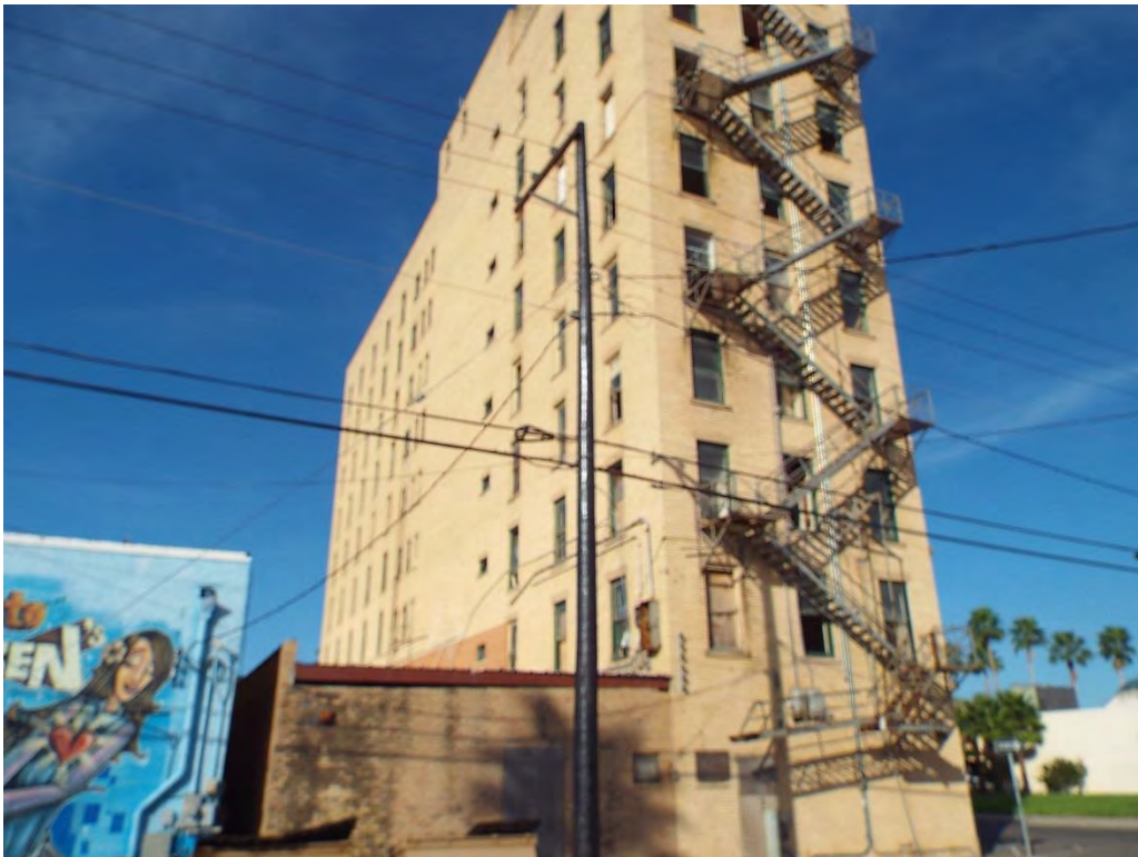
Building façade – south west elevation.
