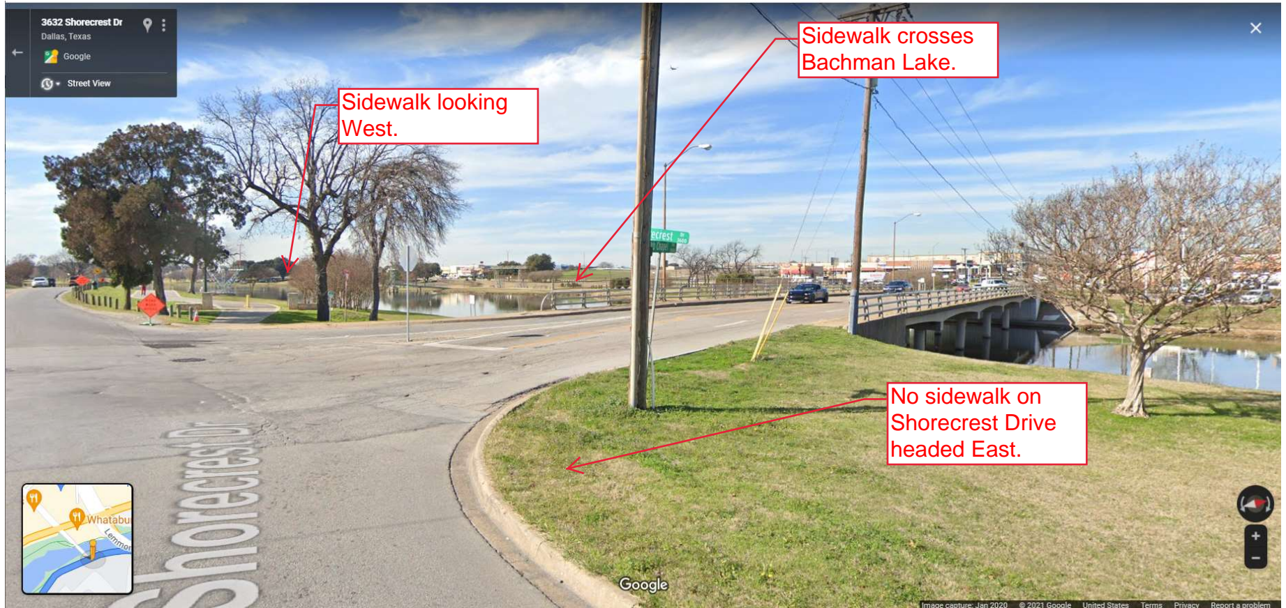
Looking west shows end of sidewalk.
