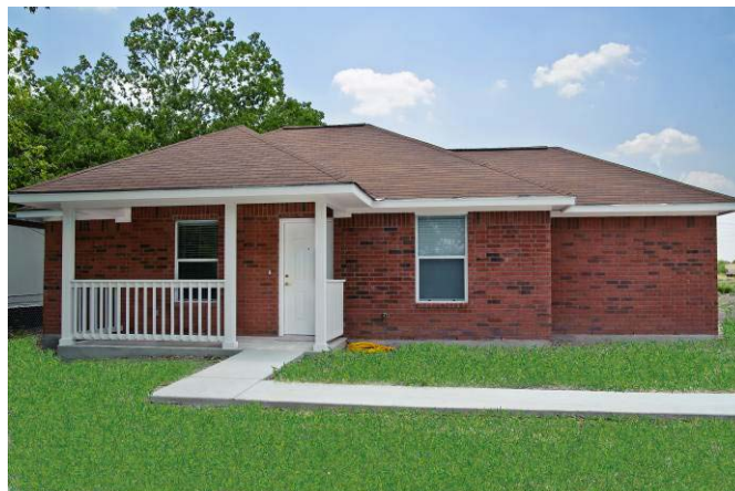
HOME's Homeowner Rehabilitation Assistance Program helps replace homes that have become uninhabitable.
